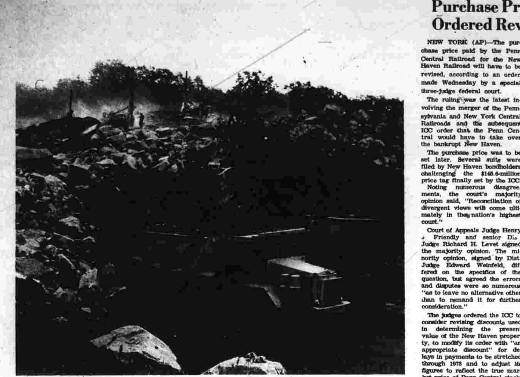
One Construction Problem of Rt. 6 Relocation
